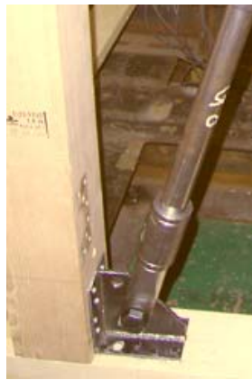
Picture 3. A fastener installed to the corner of wood frame
