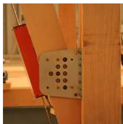
Picture 2: New brace fastener installed at the end of a brace
